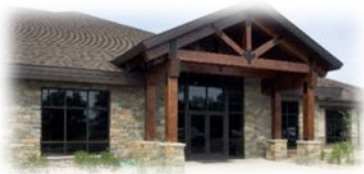
Example Portico/Covered Entry with Wood Columns - Kennedvtimber.com/au
